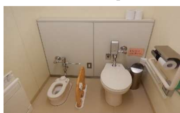
Family bathroom includes a regular size toilet with toddler size toilet
