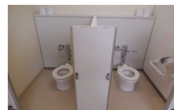
Toilets for toddler
