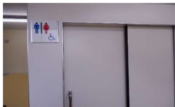
Handicap accessible multipurpose bathroom
